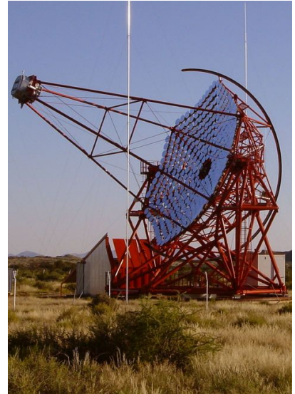
Figure 1.1: The photograph shows one of the H.E.S.S. telescopes with its mirrors mounted on the support structure and its imaging light detector held by four arms.
