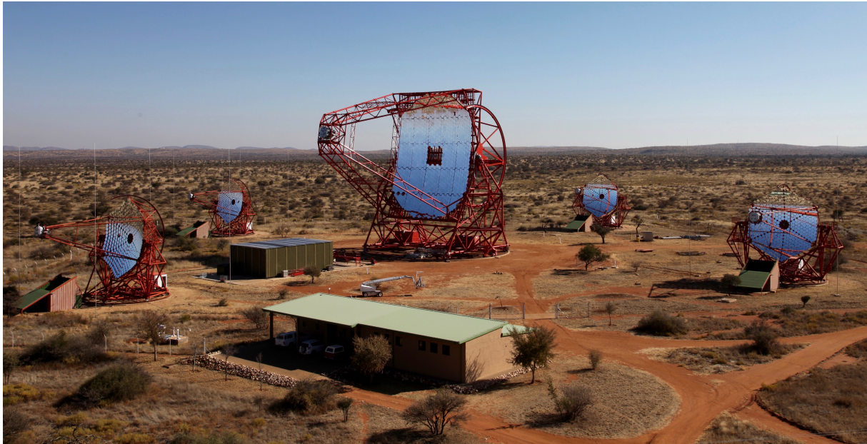
Figure 2.13.: View of the full H.E.S.S. array with the four 12 m telescopes and the single 28 m H.E.S.S. II telescope [21]
