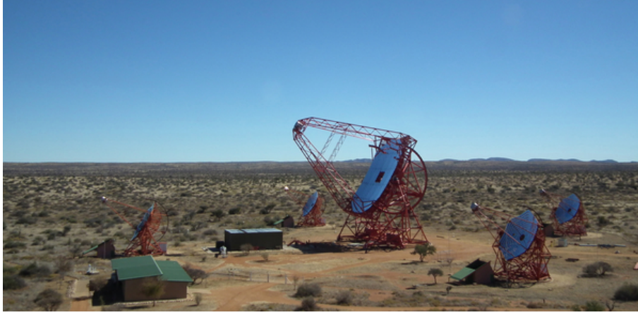
Figure 1.2: The H.E.S.S. telescope array with all five telescopes. Four small telescopes in a square formation with the larger telescope in the middle.
