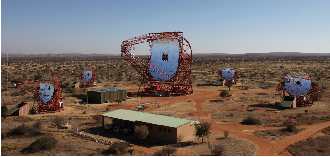
Figure 3.0.1: View of the full H.E.S.S. array with the four 12 m telescopes and the 28 m H.E.S.S. II telescope. [23]
