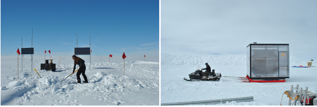
Figure 4.8: Left: In-field deployment of the first RNO-G station (Amaroq). Two solar panels are installed at the center of the station, pointing towards the south. All the hole positions and LPDA positions are marked by red flags. Right: Deployment shack being transported using a snowmobile.
