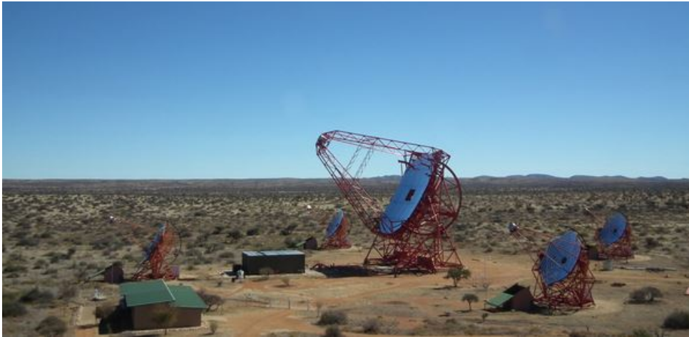
Figure 13: The H.E.S.S. telescope array in Namibia. The four 12 m telescopes are quadratically arranged and surround CT5. Figure taken from [42].
