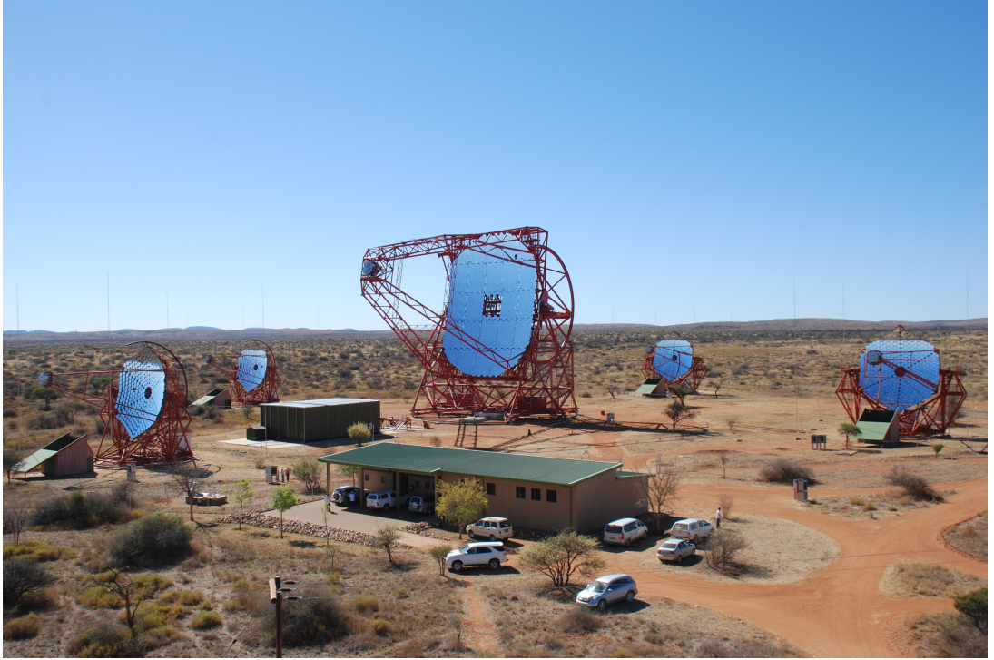
Figure 6: Photo of the H.E.S.S. site in Namibia showing its five IACTs. CT5 is positioned in the centre, and CT1-4 are located around it in a square. Taken from [26].
