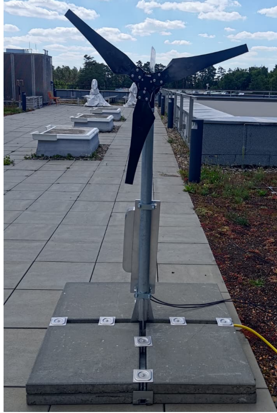
Figure 15: Horizontal-axis wind turbine installed on the roof of the ECAP. At present, the hub height of the turbine is 160 cm and is to be increased in future improvements up to 300 cm. The weight plates are already specced for the future height.
