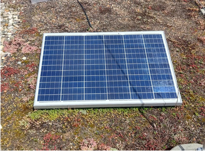
Figure 14: 100 W polycrystalline solar panel placed on the ground of the roof in front of the station.
