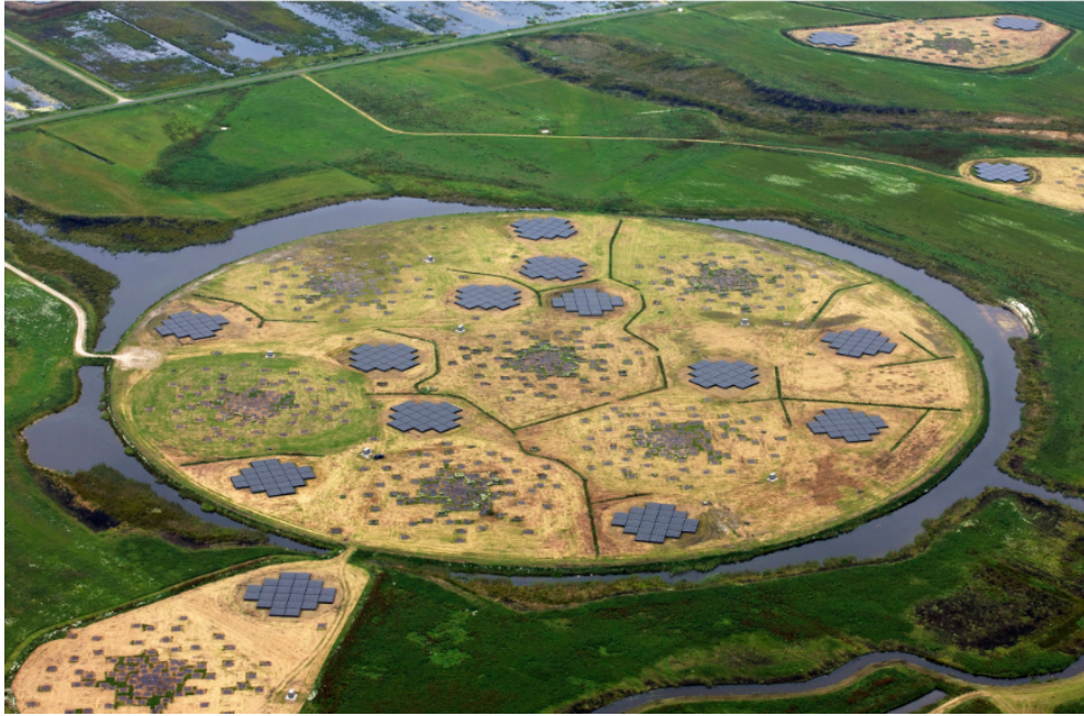
Figure 5: Picture of the Superterp, the heart of the LOFAR core. There are 6 core stations on a large circular plateau, as well as 3 additional stations visible. Figure taken from [4].
